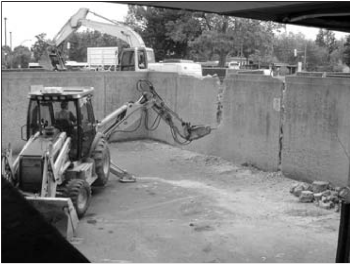
Excavating the site for the new Faculty of Dentistry building.
